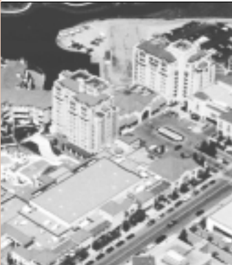
The Grand Okanagan Resort and Conference Centre, following renovations – Kelowna, B.C.
